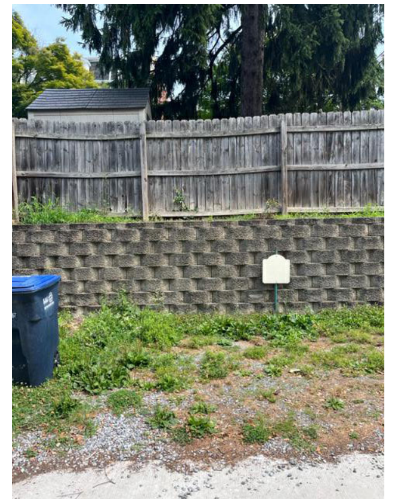
VIEW OF REAR YARD
