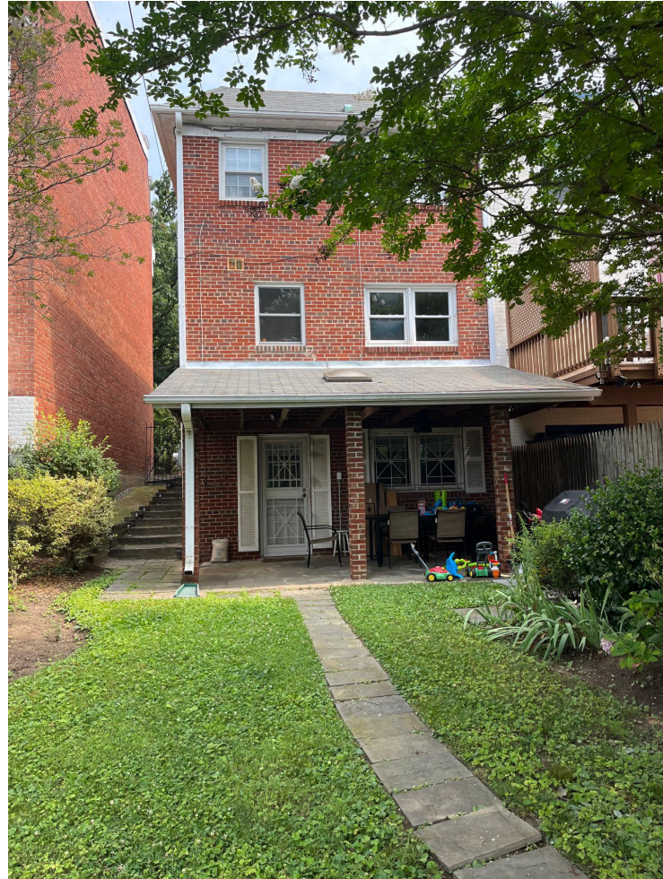
VIEW OF REAR FACADE
